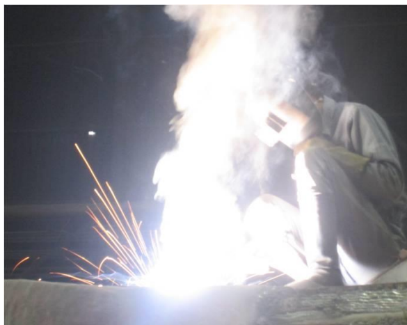
Figure 4) After designing and installing the local exhaust ventilation system
