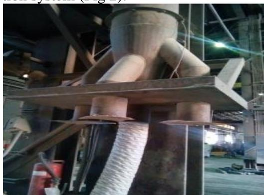
Figure 2) The central local exhaust suction system
