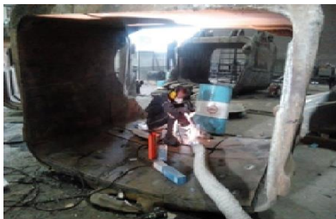
Figure 1) place where welding operations
