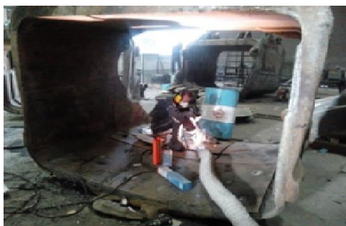
Figure 1) place where welding operations
