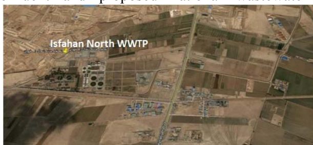
Figure 1) Landscape of Isfahan's North WWTP Land.
